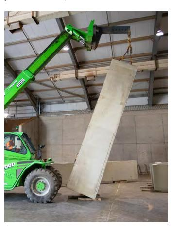
**8** Once vertical, lift the Alfabloc up sufficiently to allow the removal of the wooden bearers.
