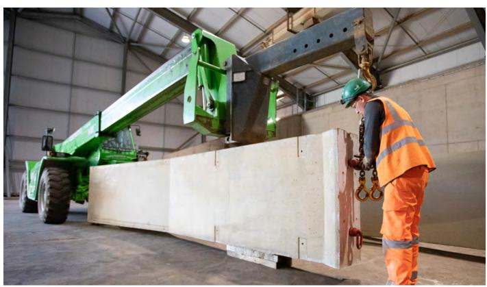
Once the chains are safely secured begin to slowly raise the boom to get the Alfabloc into an upright position.
