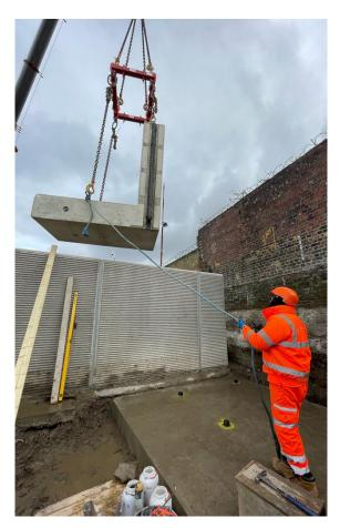
Manholes were installed for drainage, followed by backfilling with cohesive material to the top of the L wall. In order to tie in the precast walls with the existing brick wall, mass concrete with nominal reinforcement was installed for crack control.
