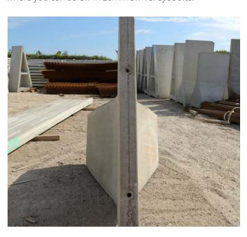
**2** Corner units are delivered lying flat and will need to be unloaded from the lorry and then stood upright before use. Place the corner unit on blocks of wood to make it easier to stand the unit up and to reduce damage to the edges of the unit.
