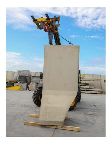
**11** Ensure the surface where the Taperblocs are going to be installed is level (this is to ensure there are no gaps in between the units when they have been installed).
