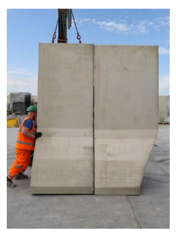
**13** If the ground is not level you may find that the units have a gap in between them. If this is the case, use packers or shrims underneath the units until they are
