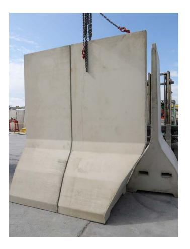
**18** Adjust the position of the Taperbloc to ensure a tight fit.
