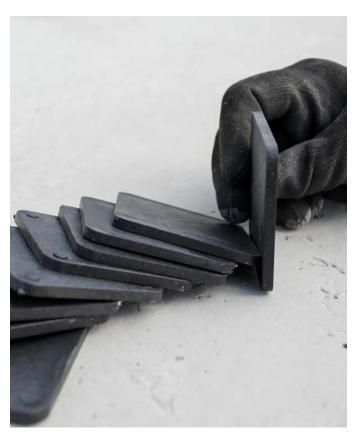
**16** To make the other corner of the wall, position the next Taperbloc at right angles into the corner unit.
