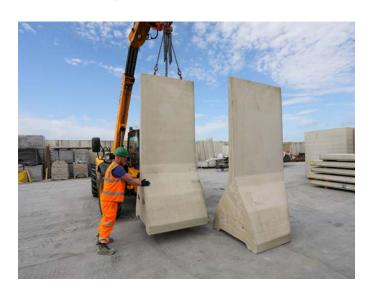
**10** Before removing the lifting chains, lift the Taperbloc up slightly and then remove the battens of wood.
