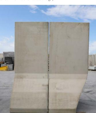
**15** Place the packers underneath the Taperblocs until the units are level.
