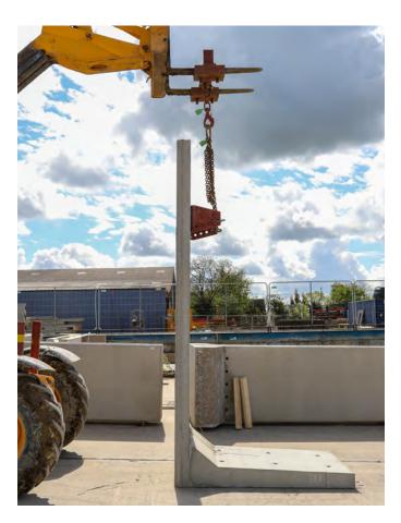
**12** If required holes can be drilled in the ground beneath the L-bloc (through the 4 holes in the L-bloc foot) to allow threaded fixing bars to be used to hold the L-bloc in position.
