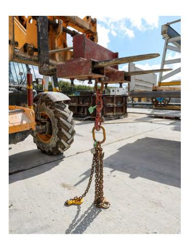
**7** Lift L-bloc slowly, balancing the weight on the heel of the L-bloc.
