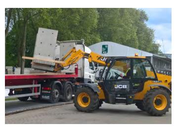
**4** Attach lifting brackets to flat surfaces of the L-bloc using countersunk bolts proved in the 4 pre-threaded holes in the L-blocs.
