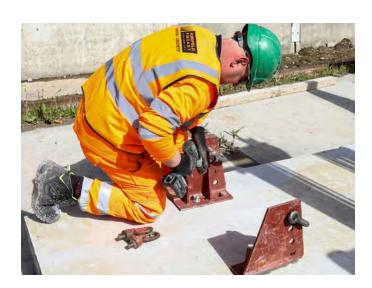
**5** Attach a lifting chain or lifting straps to the lifting brackets using D-links. Ensure that the two sides of the chain/straps are of equal length and securely fastened, to ensure a level and safe lift.
