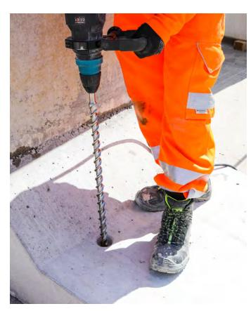
These holes should be filled with resin prior to insertion of fixing bars.
