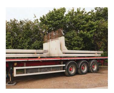
**3** The wooden batons used to separate the L-blocs on the vehicle should be placed on a suitable flat surface and used to sit the L-bloc on prior to lifting the bloc upright.
