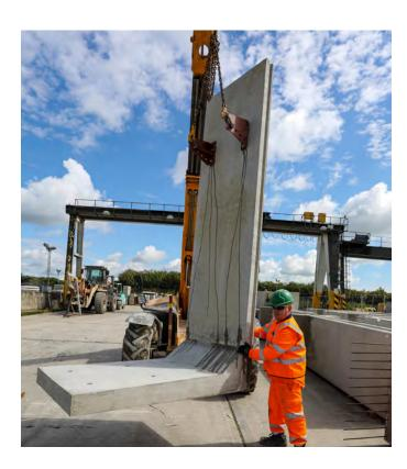
**11** Remove the lifting brackets and attach to next L-bloc.
