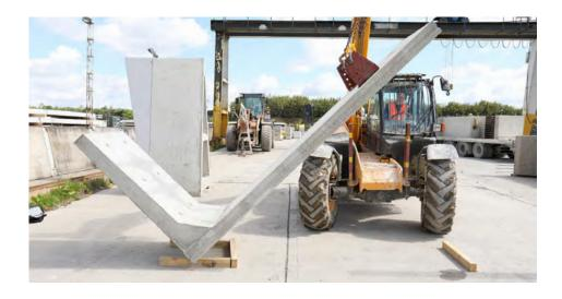
**9** Once the L-bloc is upright, it can be lifted clear of the ground and transported to its final position.
