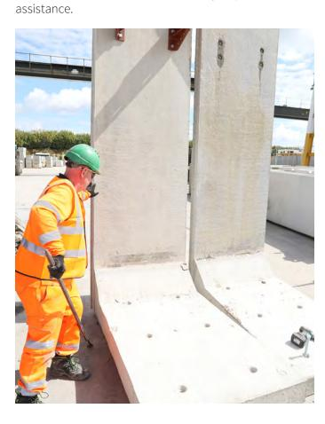
Repeat process for subsequent L-blocs. When positioning an L-bloc locate the tongue of the suspended block into the channel in the side of the installed bloc whilst the new bloc is still above ground level.
