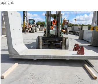
**2** L-blocs should be unloaded using a suitable fork-lift truck or telehandler.
