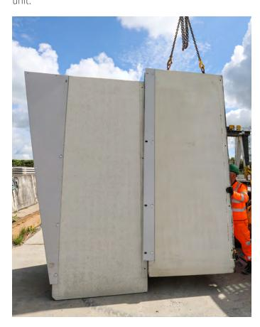
**10** Align the Alfabloc with the previously installed unit.
