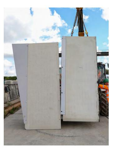
**12** Once in position lower the Alfabloc into place so that the connecting straps fit securely over the installed unit
