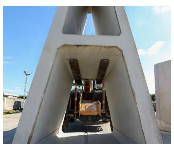
**5** If creating a 3 walled bay of Alfablocs, start in the corner and use the optional steel corner section. This allows Alfablocs to be placed at right angles to one another forming a secure sealed corner.
