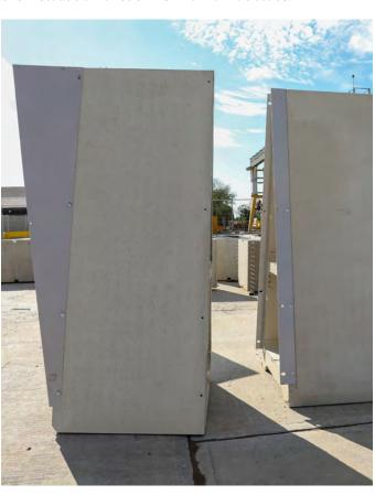
**6** Alfablocs fitted with corner sections are moved into position the same way as normal blocks fitted with connecting straps.
