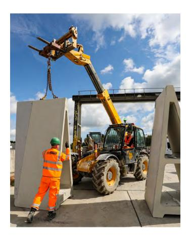
8 Attach the lifting chains to the top of the Alfabloc.
