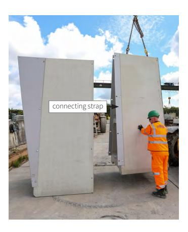
**11** Lift the Alfabloc approximately 450mm from ground level to enable you to lower it into place over the installed unit.
