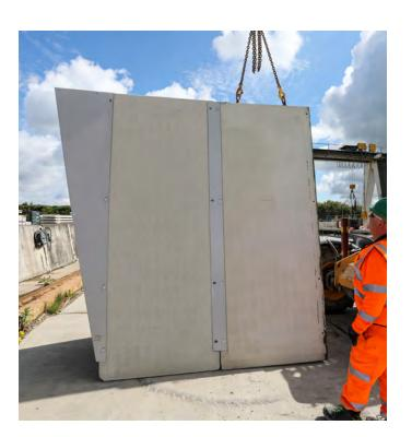
To secure Alfablocs in place, first loosen the blots in the 2 connecting straps of the freshly installed unit.
