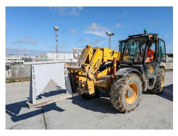
**4** 3.05m and 3.65m Alfablocs are designed to be lifted using the horizontal cross member, 1.4m above the base of the Alfabloc, and therefore no attachment is required.
